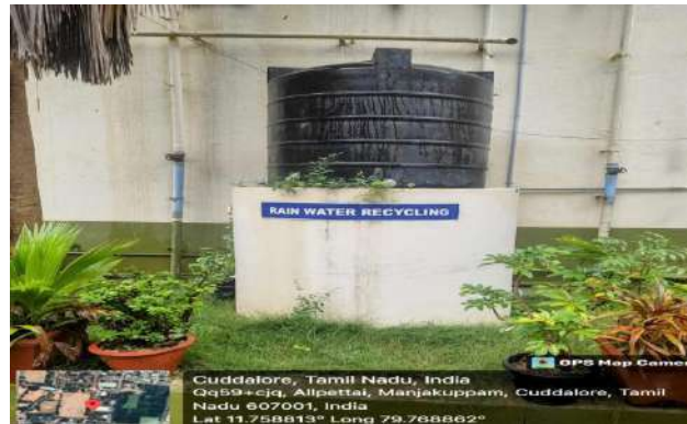
Rain Water Harvesting Tank
