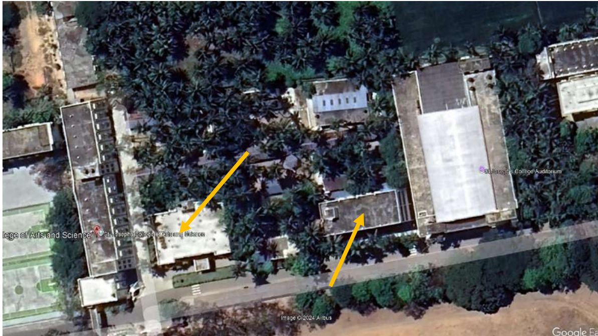
Google Map Showing the Roof Top Solar Panels That's Installed
