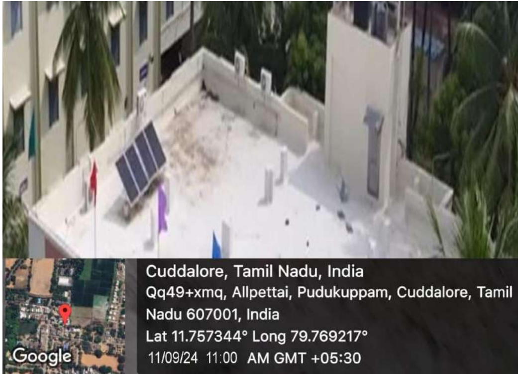
Solar Panels Used For Harnessing Solar Energy
