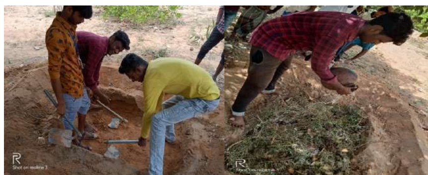
Construction of Vermicomposting pits by Enviro club volunteers
